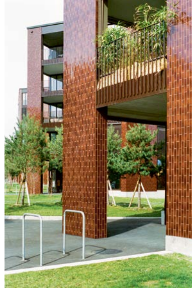
5.11 Ceramic tile facade, Katzenbach IV, 2020
