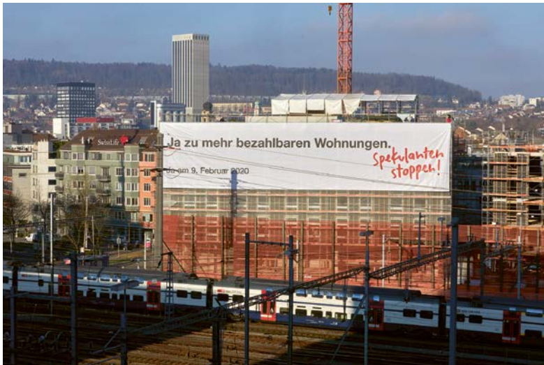
2.14 Banner on the Zollhaus construction site for the popular initiative More Affordable Housing, 2020
