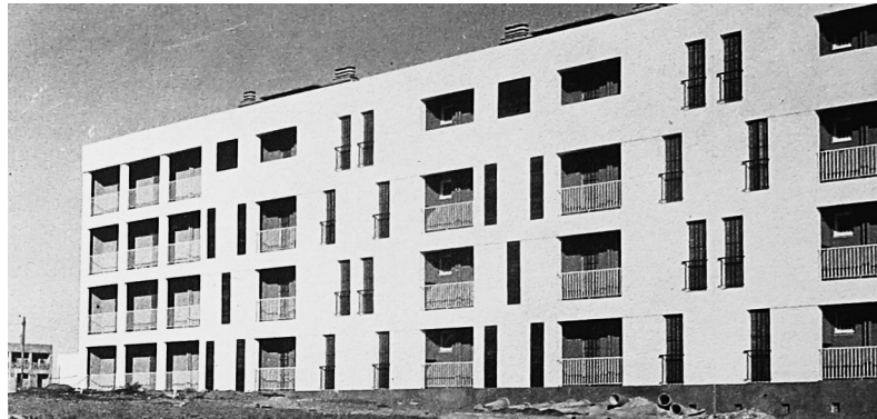
Figs. 64a, 64b, 64c Housing units designed by Daure and Béri in Rocher Noir
