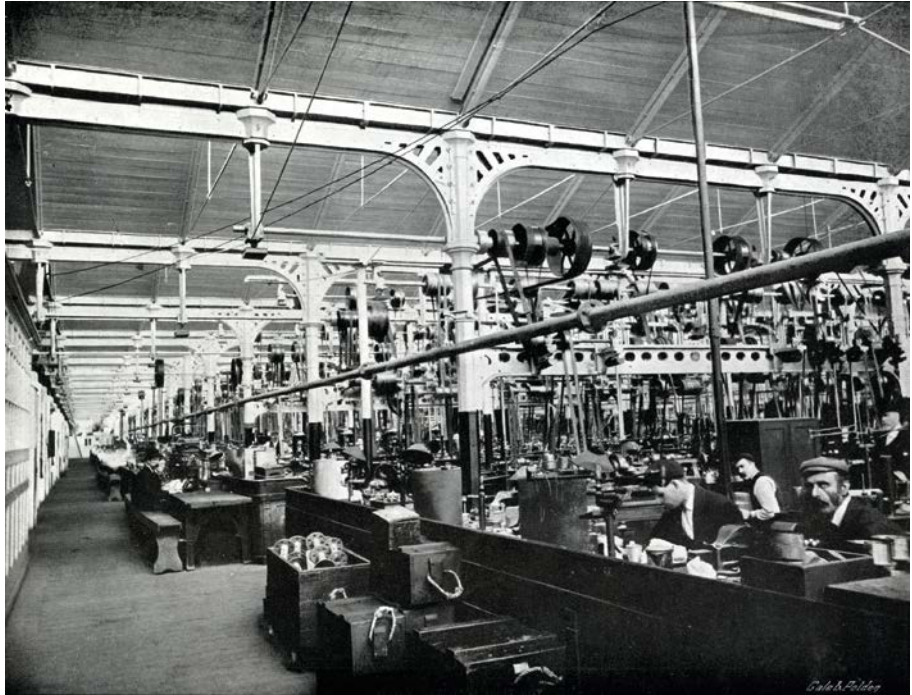
Figure 6. Thomas Bernard Collinson and Gottfried Semper, machine shop, Royal Laboratory, Woolwich Arsenal, London, 1854, as shown here in use for ammunition production in 1914 (Courtesy of the Greenwich Heritage Centre).
